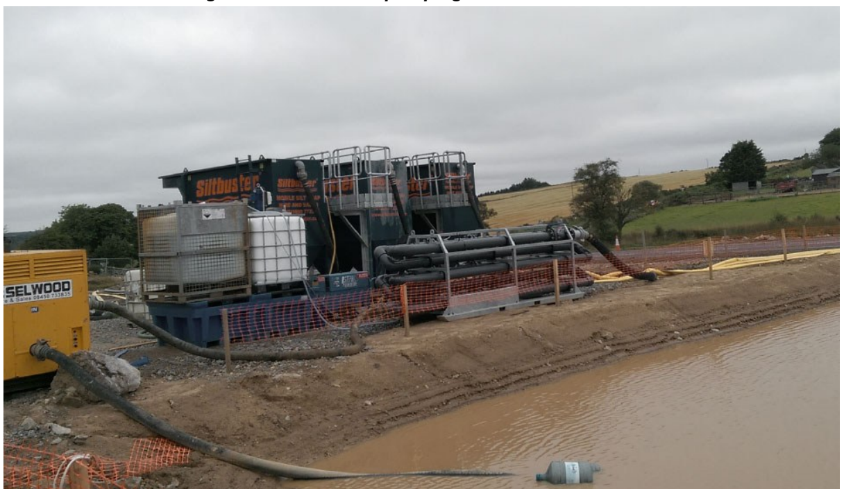
Plate 7: Settlement lagoon and Siltbuster pumping out water for treatment
