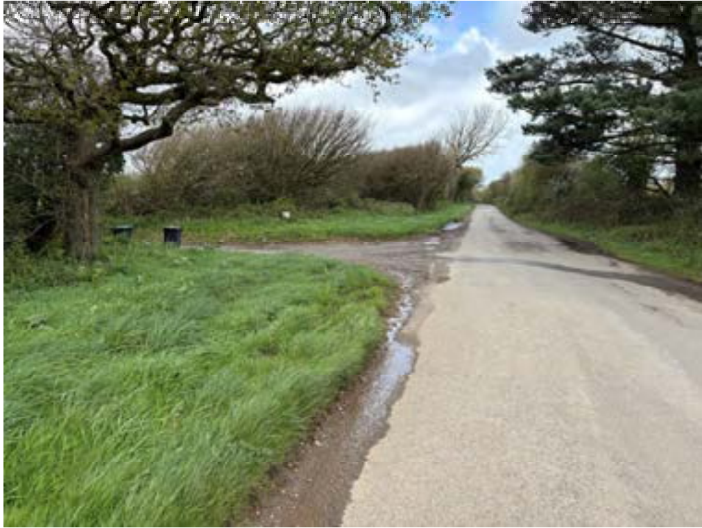
Image 2.4 – Principal Site Access (Left of Image) from White Cross Road
